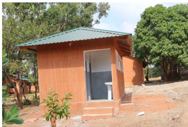
Image 2: part of the infrastructure built at the Mabeco gate as part of the improvement and construction of support infrastructures
